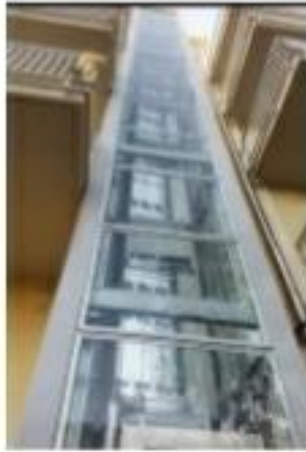
EXTERNAL GLASS LIFT SHAFT
