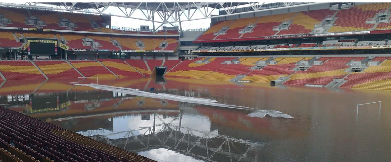
Figure 19: Lang Park (Suncorp Stadium) in Brisbane submerged after intense rainfall and floods in January 2011. For each 1°C rise in global average temperature, the atmosphere can hold approximately 7 percent more moisture, in turn increasing the probability of more intense rainfall events such as occurred in Brisbane in 2011.
