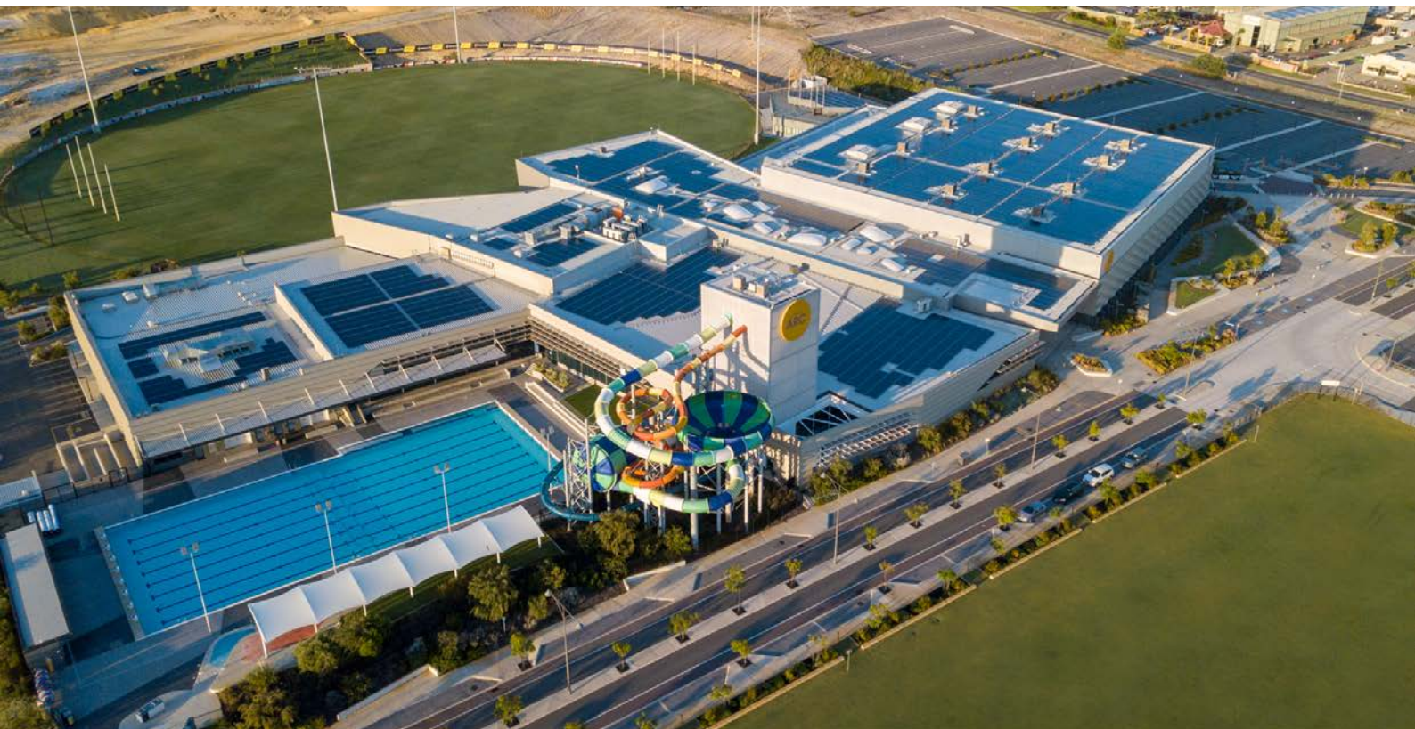
Figure 22: Cockburn Aquatic and Recreation Centre in Western Australia, which hosts one of the largest rooftop solar systems in the state.
