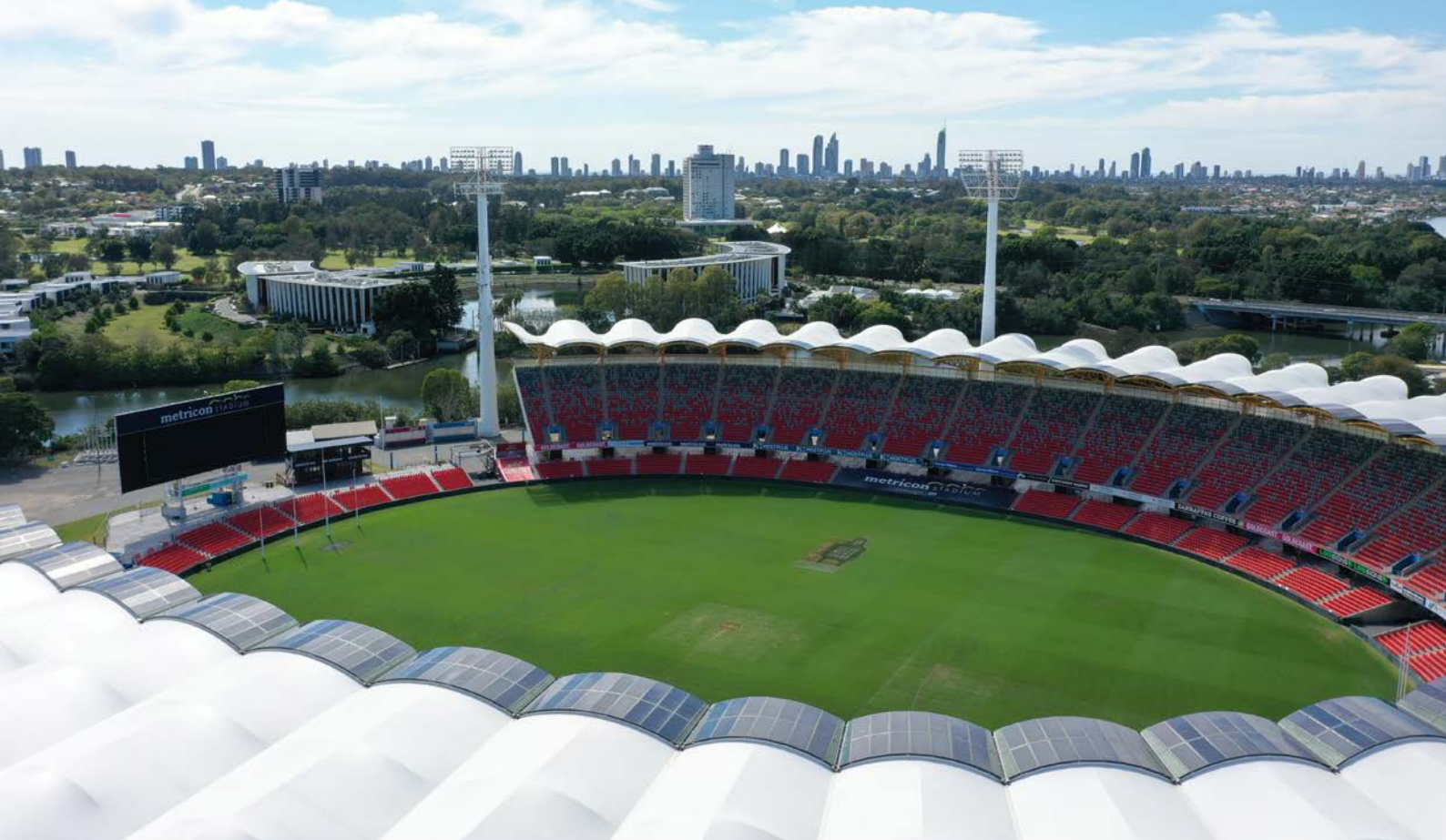
Figure 25: Metricon Stadium on the Gold Coast, with a 'solar rim' of solar panels along the inner roofline, supplying roughly 20% of the stadium's electricity.
