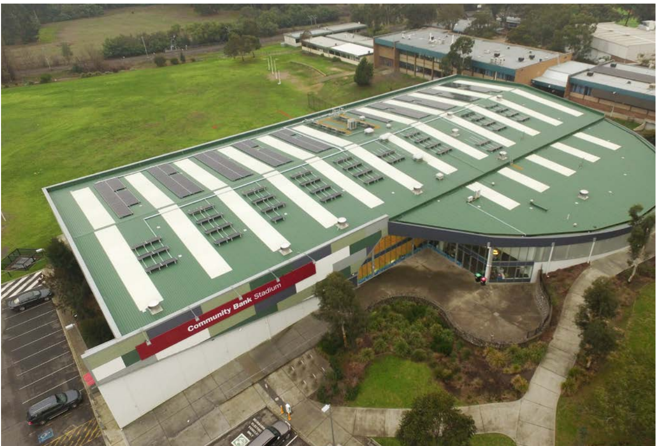
Figure 26: Nillumbik Shire Council's Hybrid Solar and Battery Off-Grid Community Stadium & Relief Centre in Victoria, which features rooftop solar, a battery system and an electric vehicle charging station.
