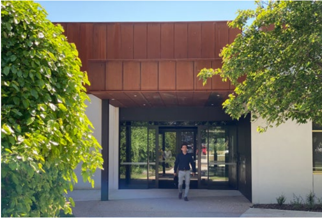
Image 5. The recently refurbished Community Centre.
