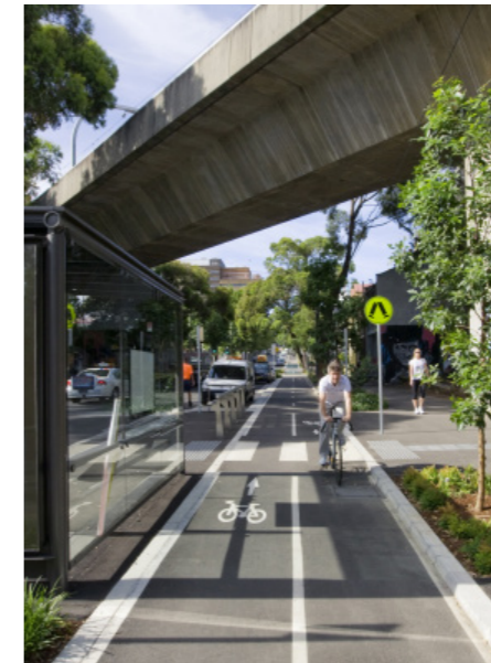
Bidirectional Separated Cycleway Bourke Street, Sydney, NSW
