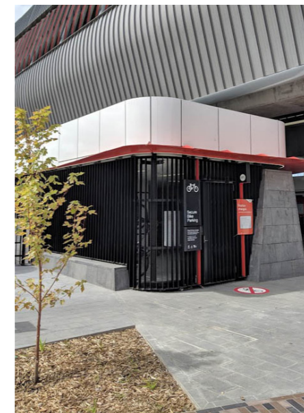
Secure Station Bicycle Storage Murrumbena, VIC
