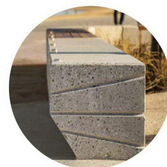
Insitu concrete seating
