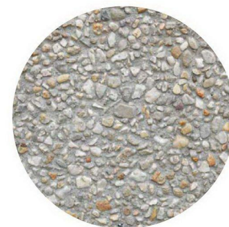
Exposed Aggregate Concrete
