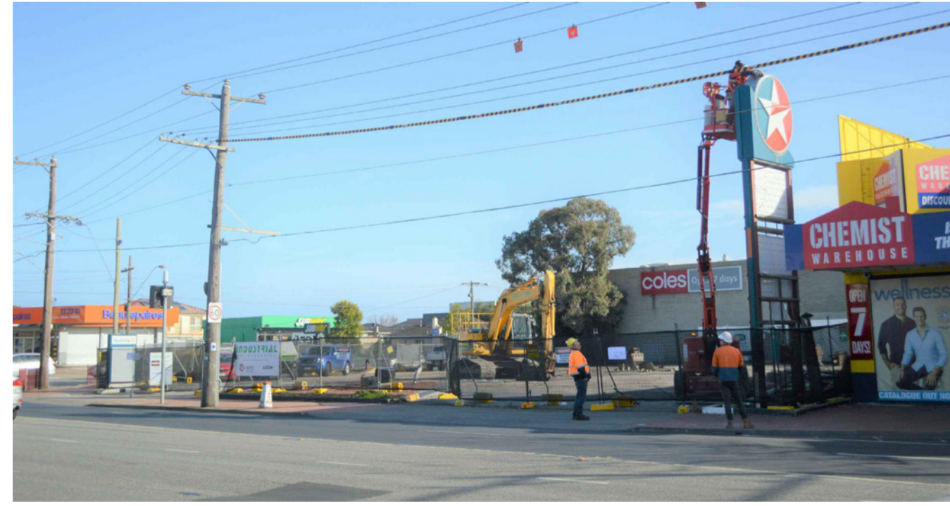
03 SITE PHOTO: VIEW FROM CLAYTON ROAD LOOKING TOWARDS SOUTH WEST NTS
