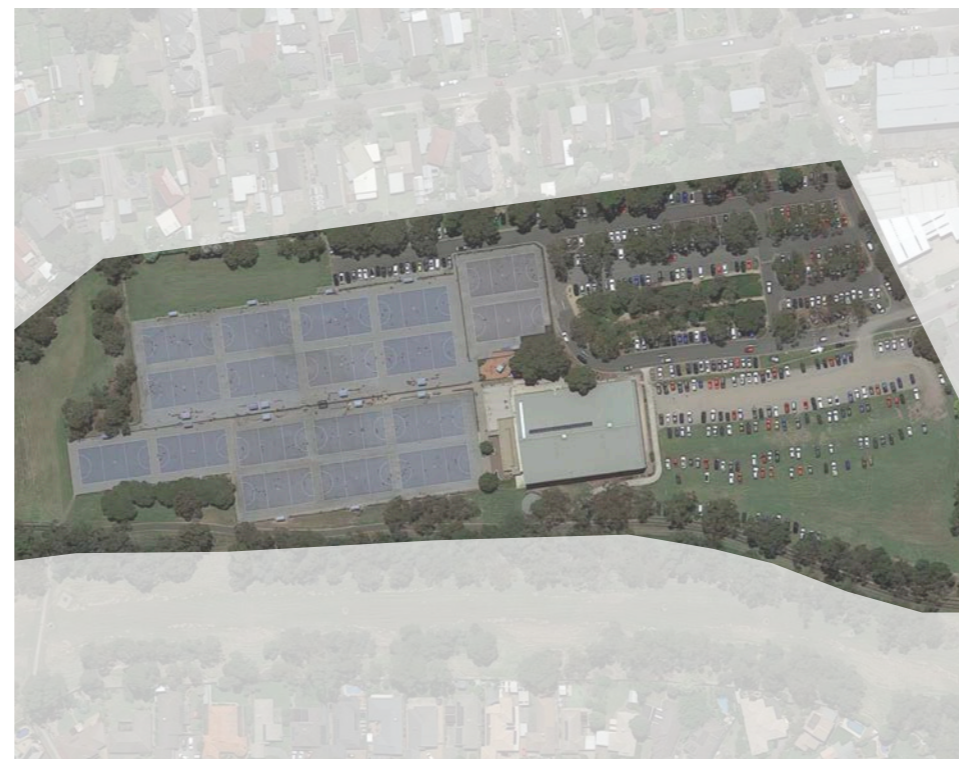
Knox Regional Netball Centre (Ferntree Gully)
