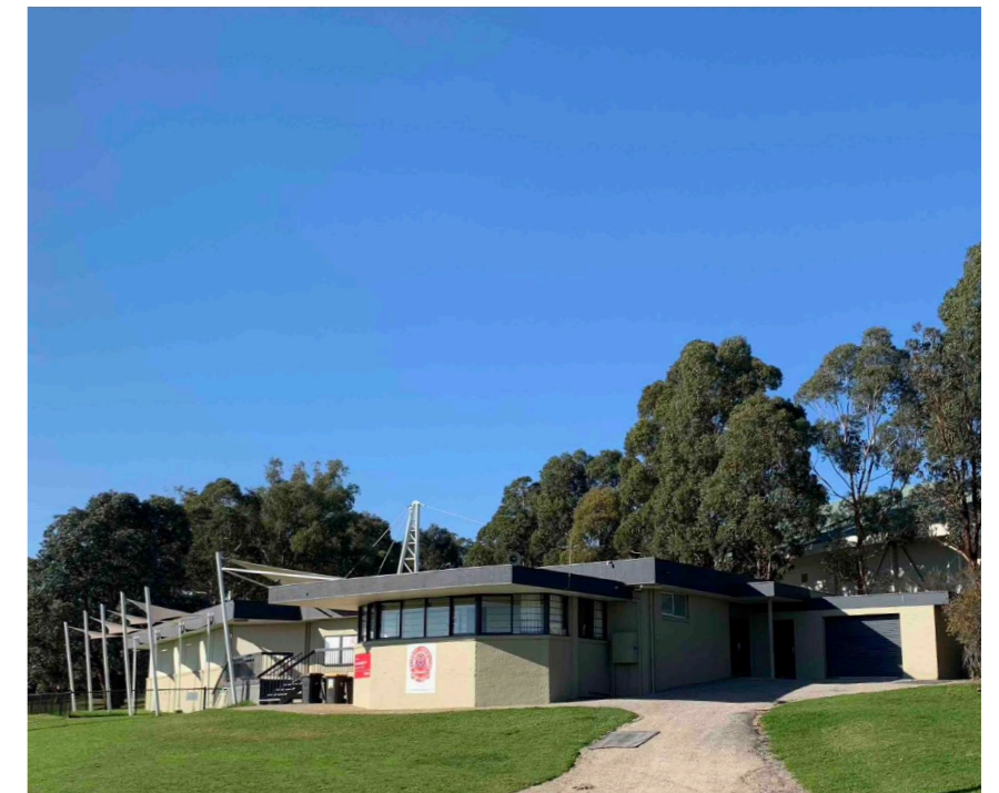
The existing softball pavilion, viewed from the north-west.
