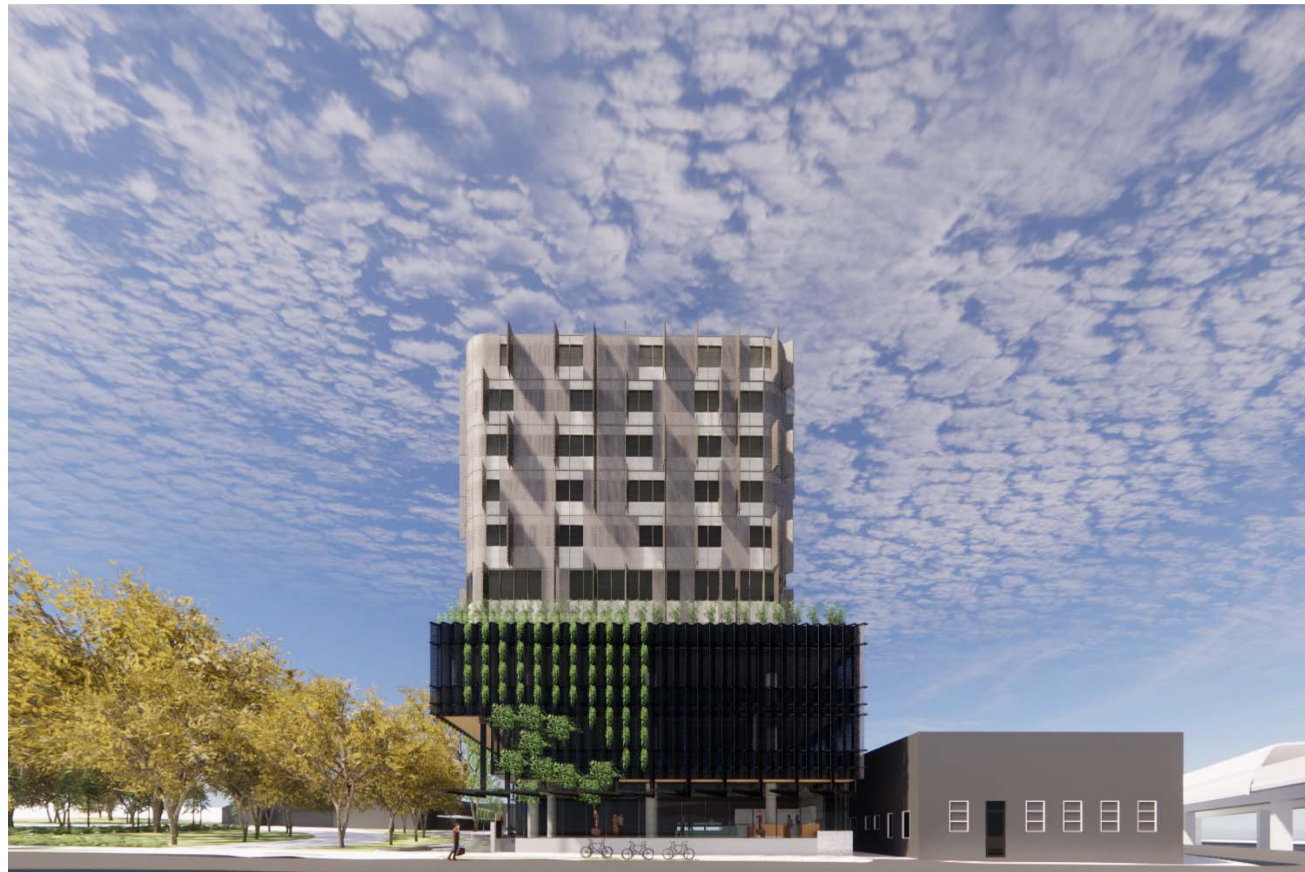
WEST FACADE PANELS PARTIALLY OPEN
