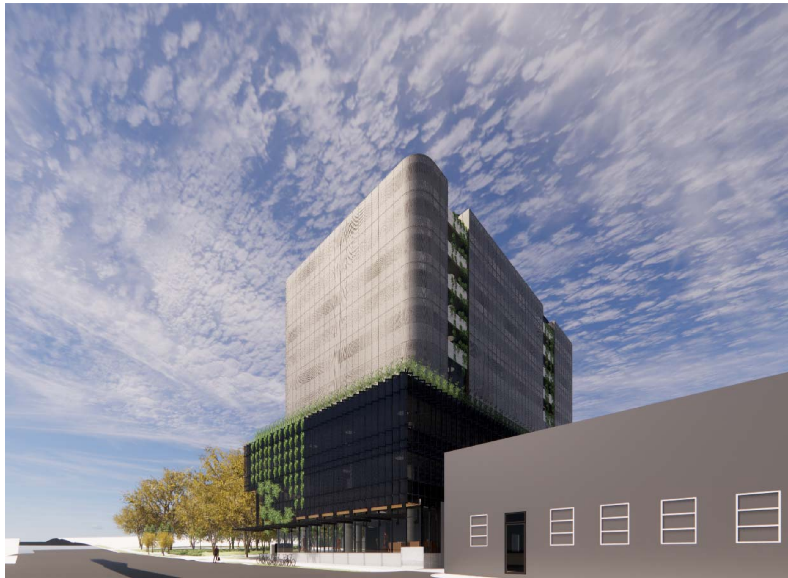
SOUTH WEST FACADE PANELS FULLY CLOSED
