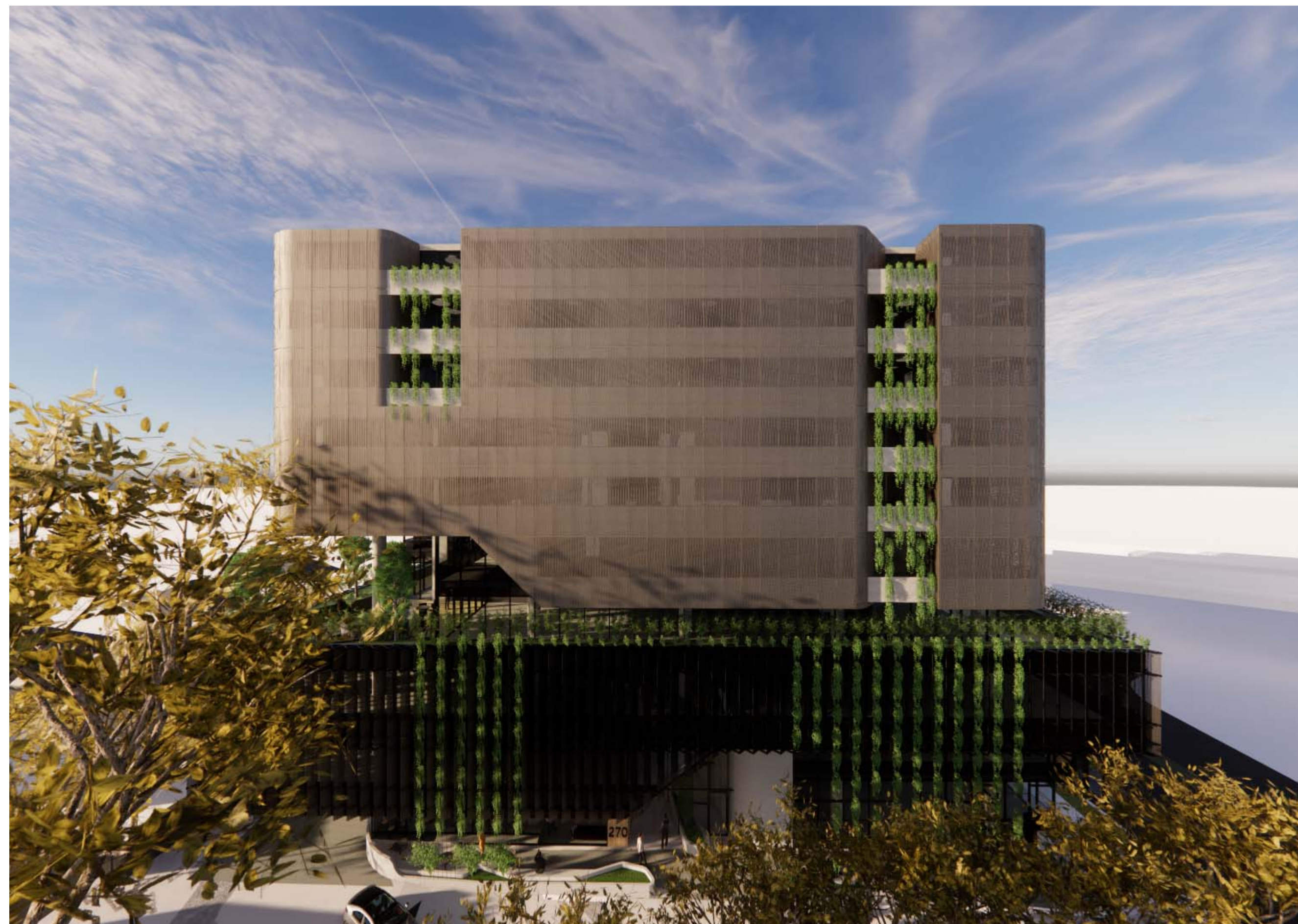
NORTH FACADE PANELS FULLY CLOSED
