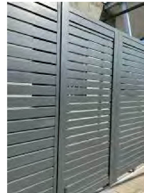
PLANT SCREEN: ALUMINIUM SLAT SCREEN
