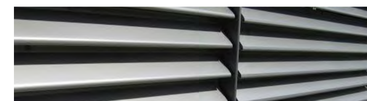
ALUMINIUM TILTED PRIVACY LOUVRES ABOVE 1.2M BALUSTRADE
