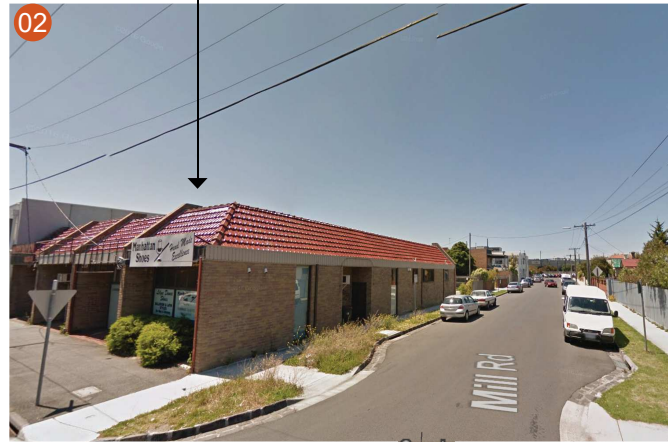
MILL ROAD / JOHNSON STREET INTERSECTION LOOKING NORTH-EAST
