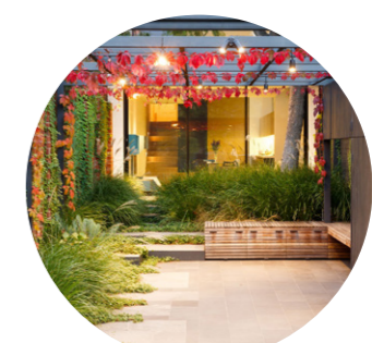
Trellis Steel with cables for climbing plants
