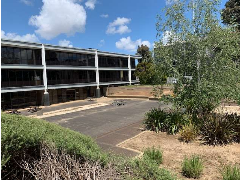
Figure 4 – Rear of BHP Building, Sunken Courtyard
