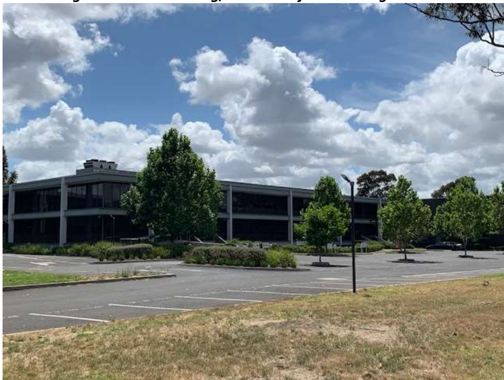
Figure 3 – BHP Building, as viewed from Wellington Road
