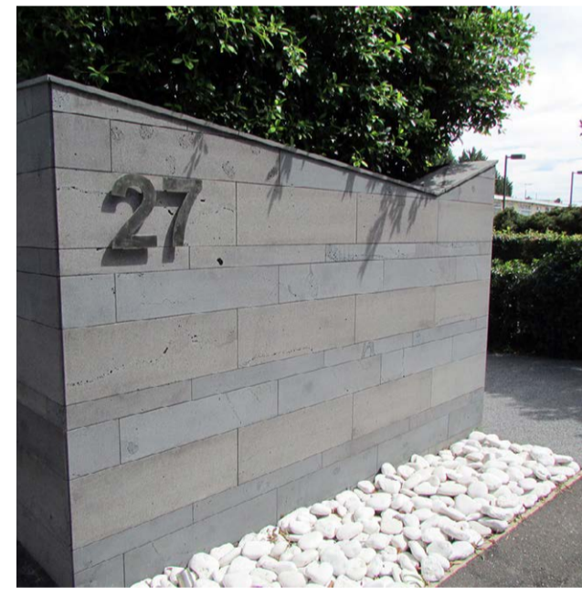
Blueastone entry gate and fence
