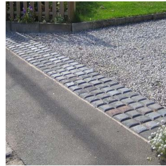
Porphyry stone rumble strip
