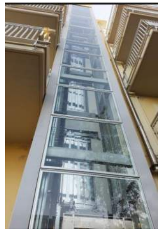
EXTERNAL GLASS LIFT SHAFT
