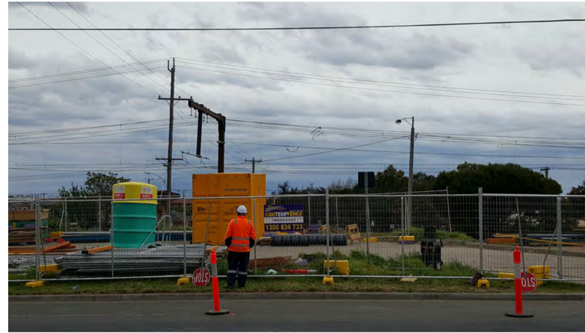
RAILWAY WORKS OPPOSITE No 179 CARINISH RD
