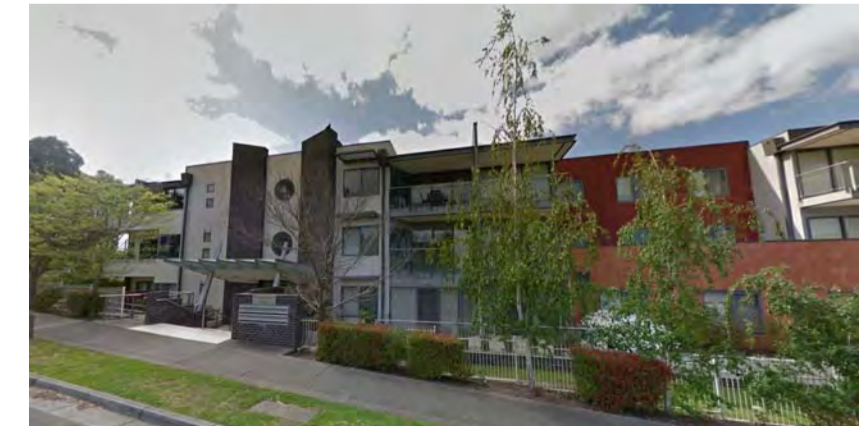
2 Blair Road Glenview Service Apartments
