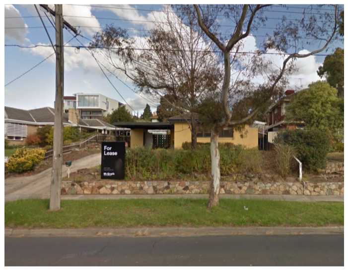
D 250 Highbury Road - Subject Site
