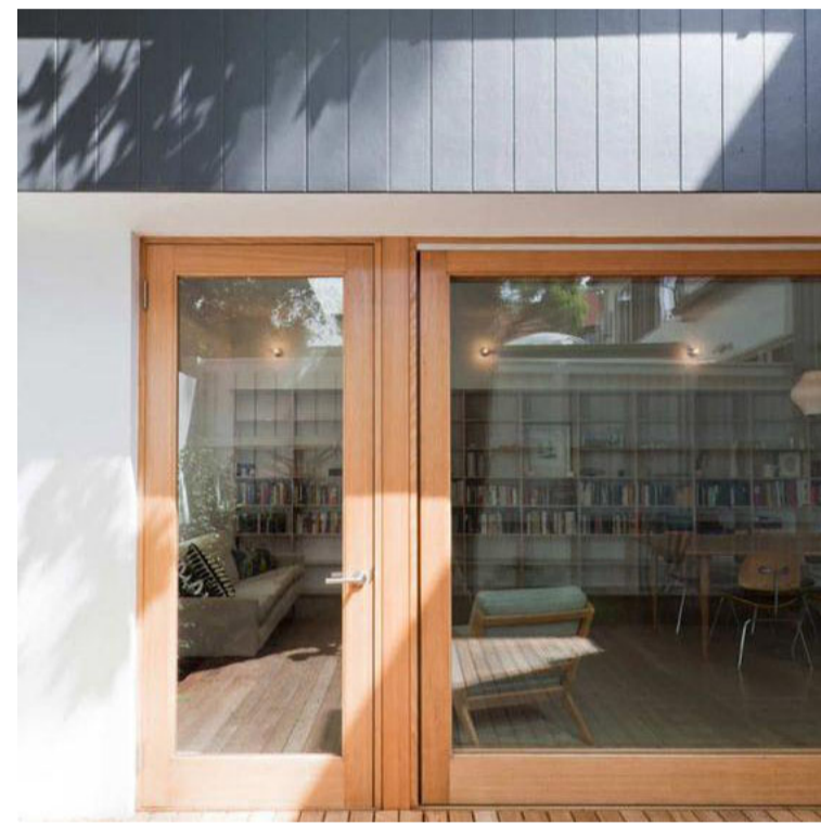
D01/D05 - TIMBER FRAMED ENTRY DOORS.
