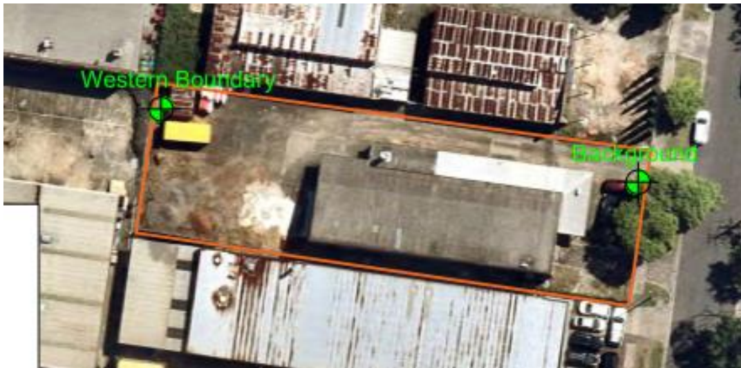
Figure 6 – Extract from site area plan included within the report prepared by Focus Environmental dated 30 November 2023
