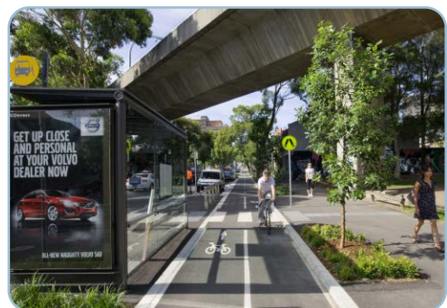
Bidirectional separated cycleway: Bourke Street, Sydney NSW
