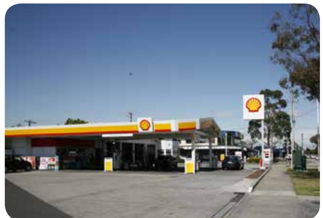
Site C - Shell Service Station
