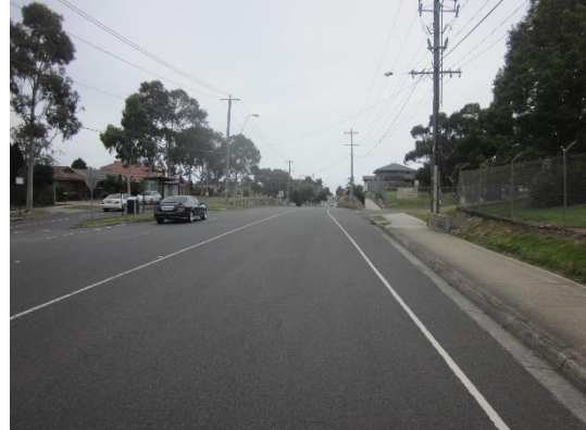
Figure 2.5: Jacksons Road (Looking South)
