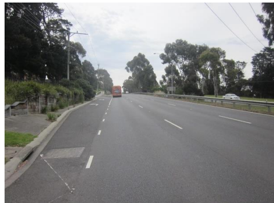
Figure 2.7: Wellington Road (Looking West)
