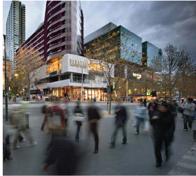
Glazed ground floors with podium built to the street edge contributes to street vitality. Tower forms set back above podium
