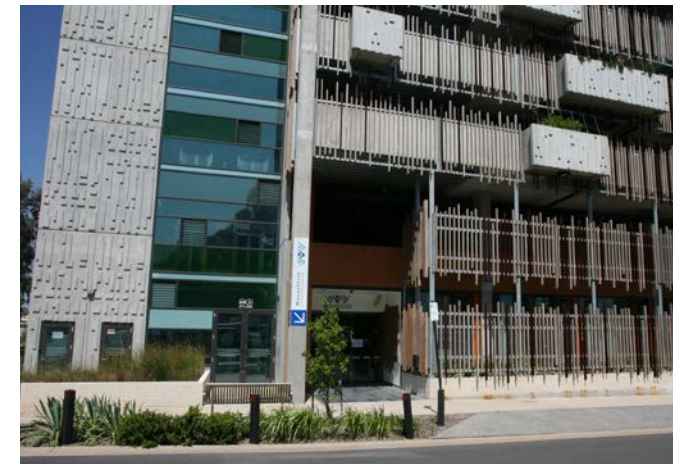
The existing Euneva Community Health Service
