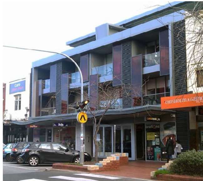
Interactive facades and glazed openings in upper podium levels provide opportunities for passive surveillance of the public realm
