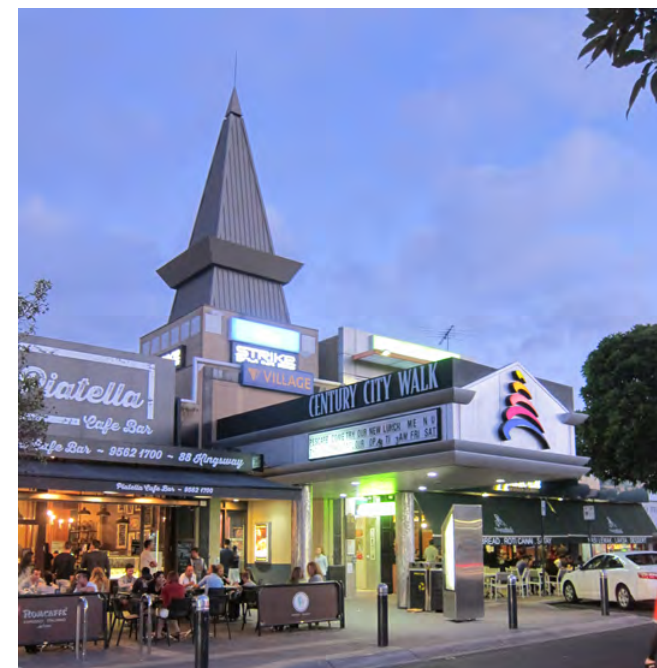
The entrance to Century City Walk in Kingsway
