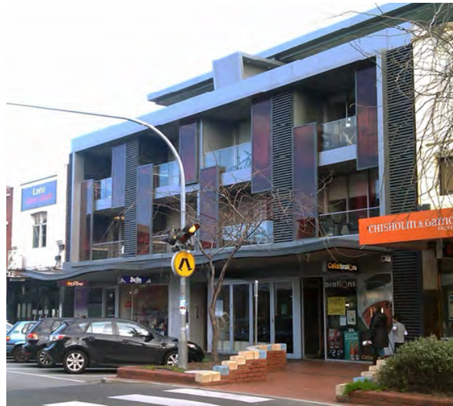
Interactive facades and glazed openings in upper podium levels provide opportunities for passive surveillance of the public realm
