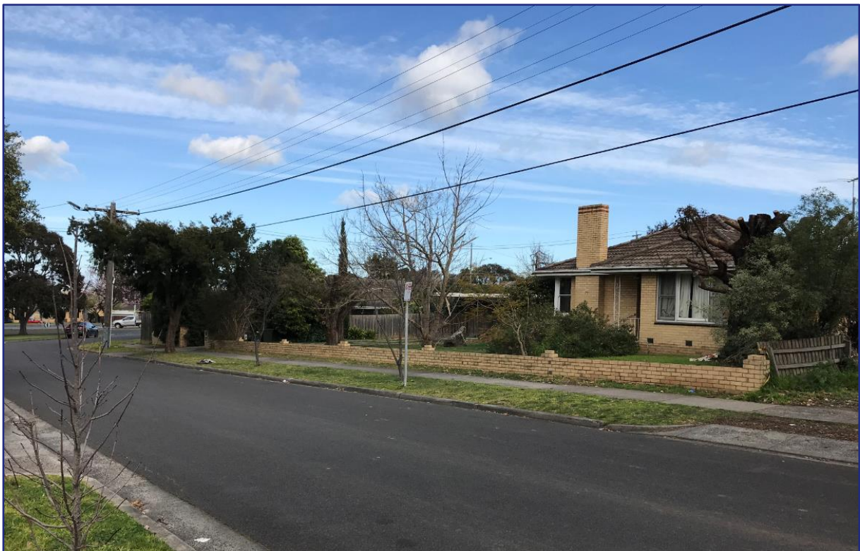
Figure 4: Subject site frontage to Beddoe Avenue (view south-west)
