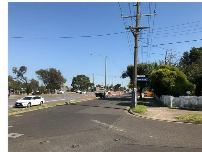
Princes Highway Service Road with Princes Highway beyond
