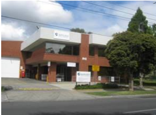
Figure 44: Stamford Road Precinct
