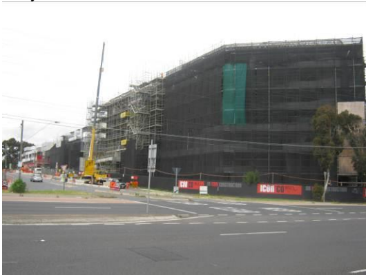
Ashwood Chadstone Gateway Project (Power Avenue)
