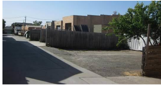
Rear laneway access for Haughton Road properties
