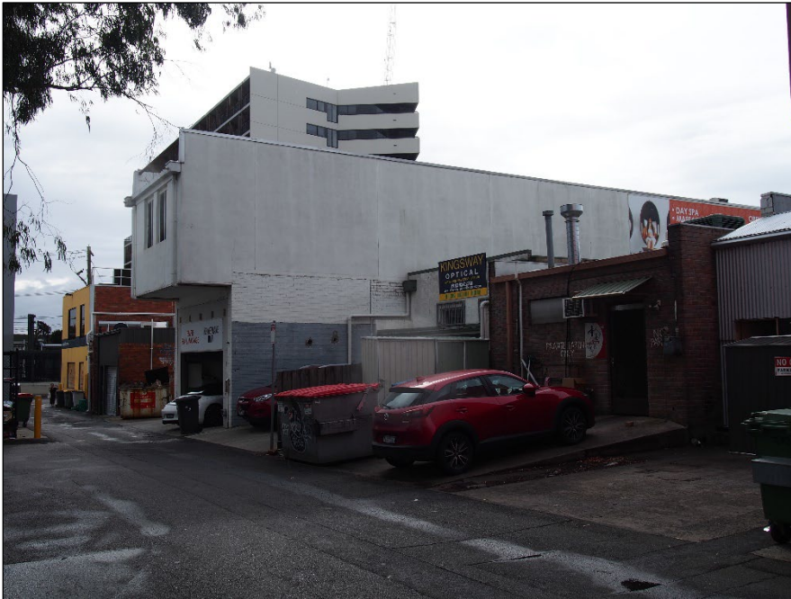
View towards the rear of the subject site from Montclair Avenue.
