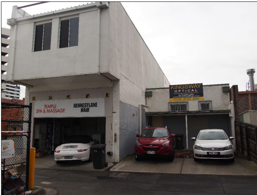
View of the rear of the subject site from within the laneway.
