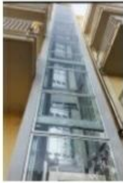
EXTERNAL GLASS LIFT SHAFT
