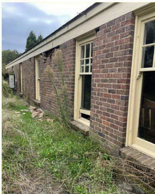
Photograph 2: Existing Dwelling on lot 1
