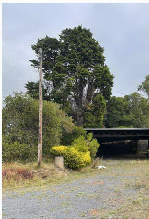
Photograph 3: Existing carport on lot 1
