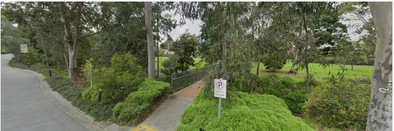
Picture 5 Image of the connection bridge, south-west of the site.
