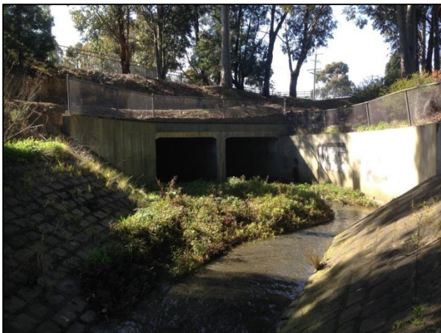
Plate 3: Culvert with highly modified banks
