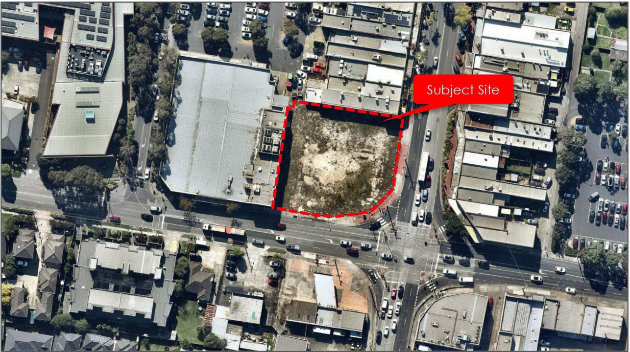
Figure 2 Site Context (24 April 2023)
