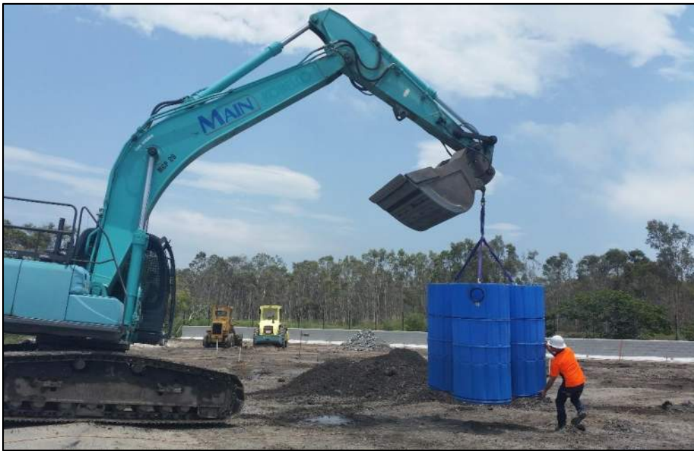
Figure 4.3: SPEL Hydrosystem (SHS.1000) installation using onsite digger
