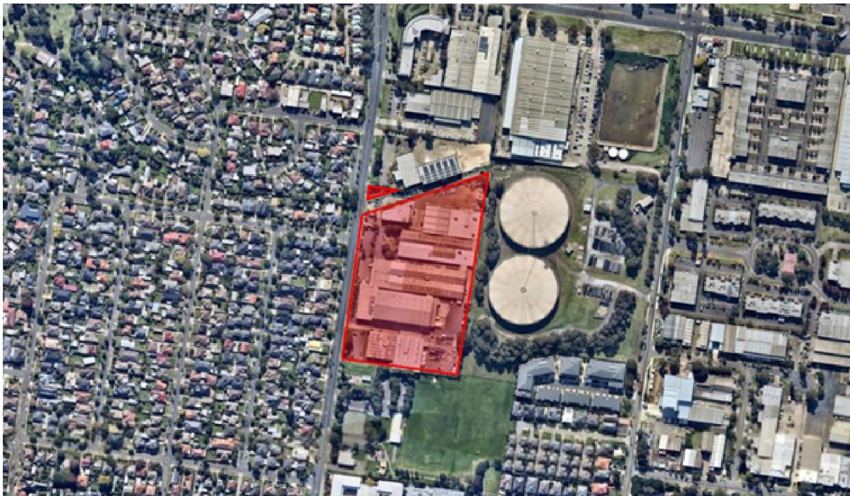
Figure 1: Aerial view of the site at 34-54 Clayton Road, Clayton, showing the approximate site boundary. (Source: Nearmap, Mark-up: WRAP Engineering)
