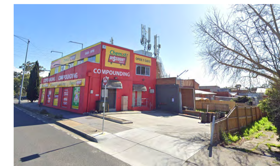
VIEW 14 - NO 545 WARRIGAL ROAD 2 STOREY BRICK COMMERCIAL
