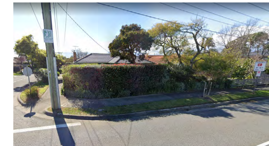
VIEW 06 - NO 35 SINGLE STOREY TILED PITCH ROOF WEATHERBOARD RESIDENCE
