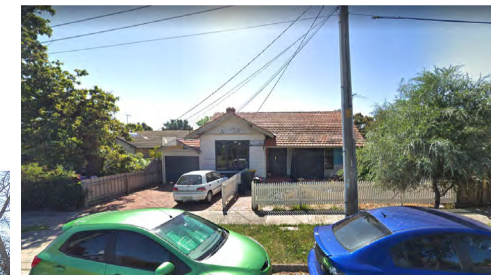
VIEW 09 - NO 6 KENNETT STREET, SINGLE STOREY TILED ROOF WEATHERBOARD RESIDENCE
