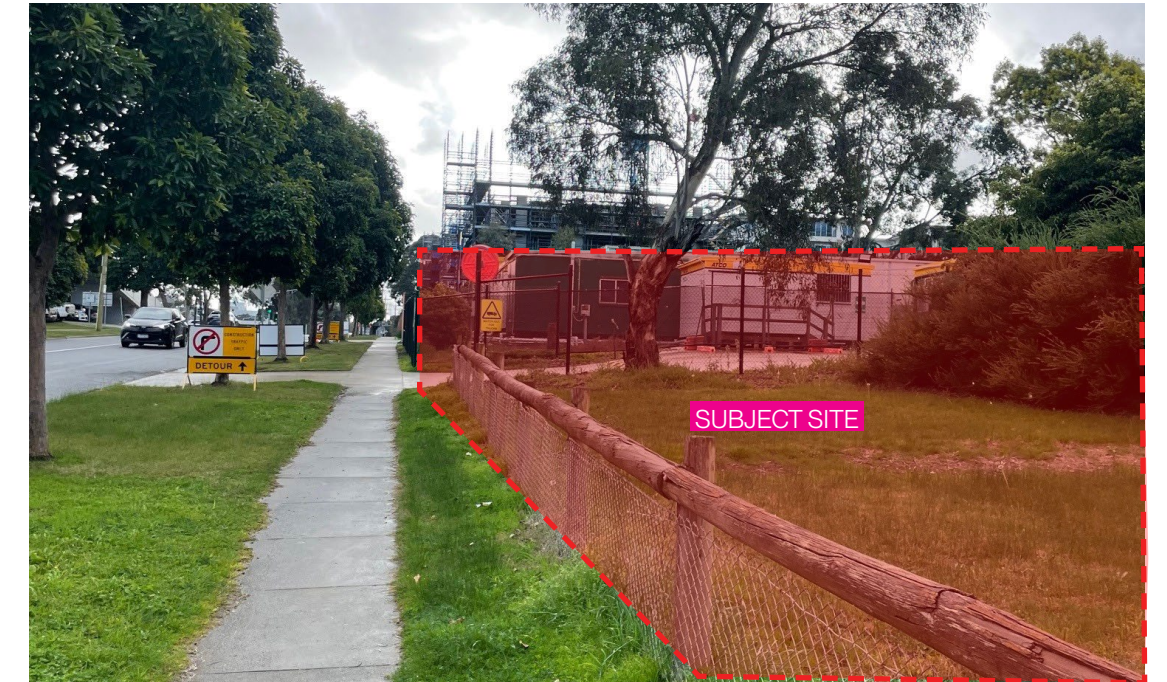
3 View along Brandon Park Drive & Academy Ave looking North East
