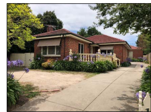
P01 View north east towards #1/194 Clayton Road.
