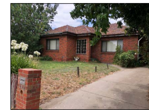
P02 View north east towards #192 Clayton Road.
