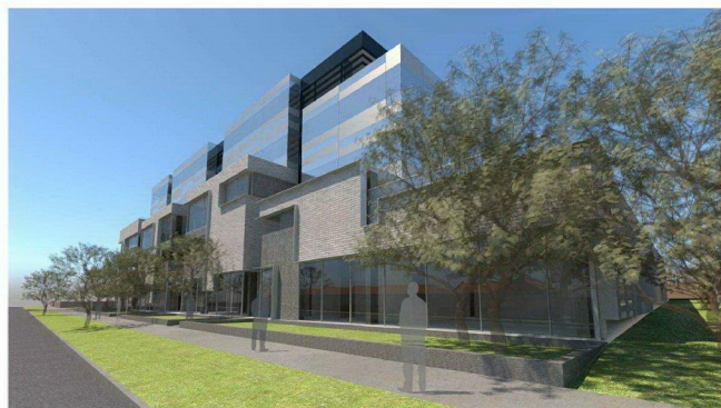
SOUTH WEST VIEW
