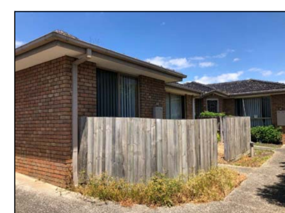
P06 View south east towards #3/2 Whitburn Street.
