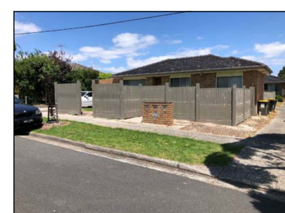
P05 View south east towards #1/2 Whitburn Street.
