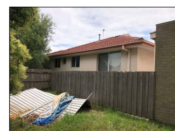
P07 View north east towards the rear of #2/1 Hourigan Avenue.
