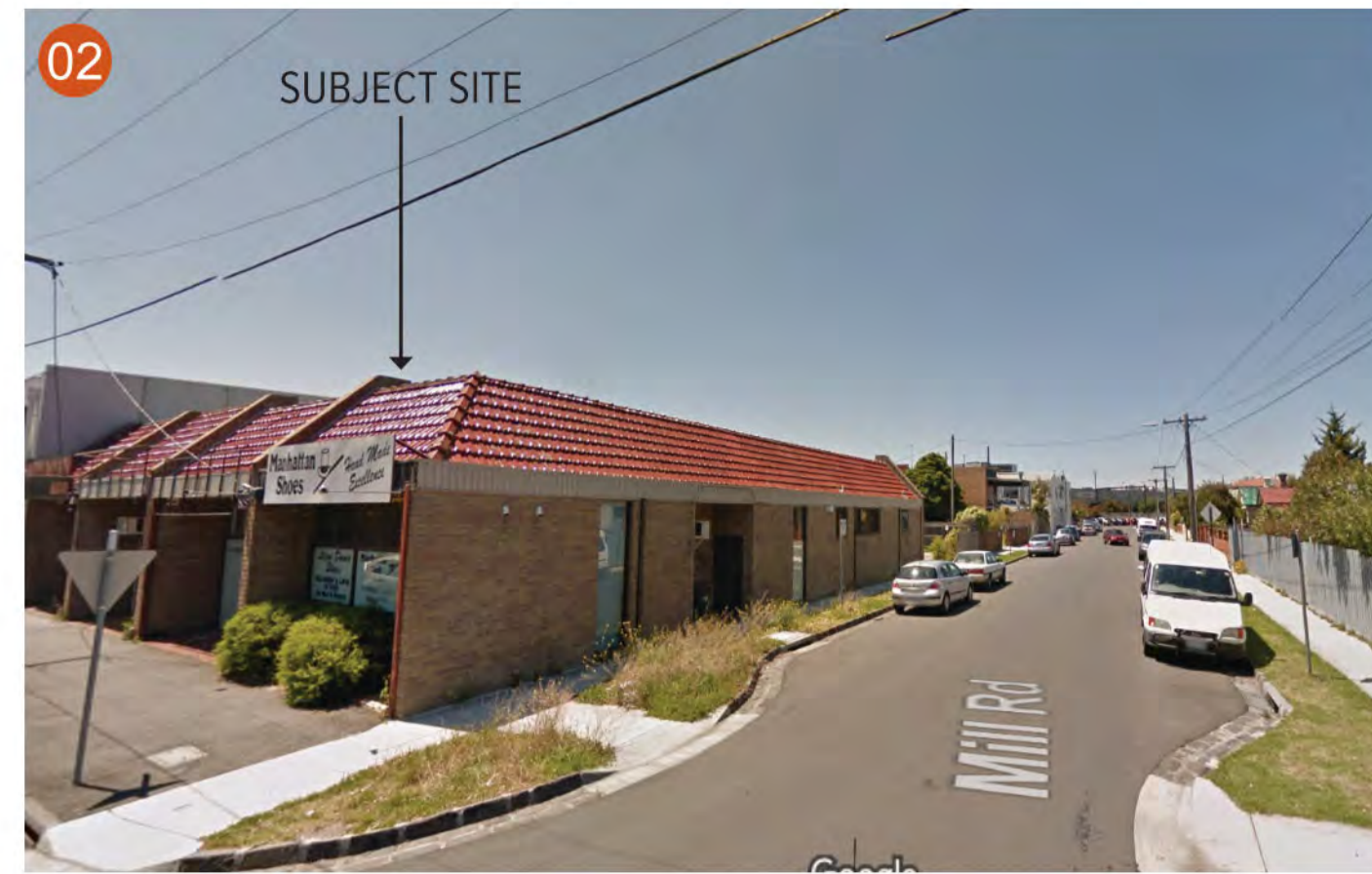
MILL ROAD / JOHNSON STREET INTERSECTION LOOKING NORTH-EAST
