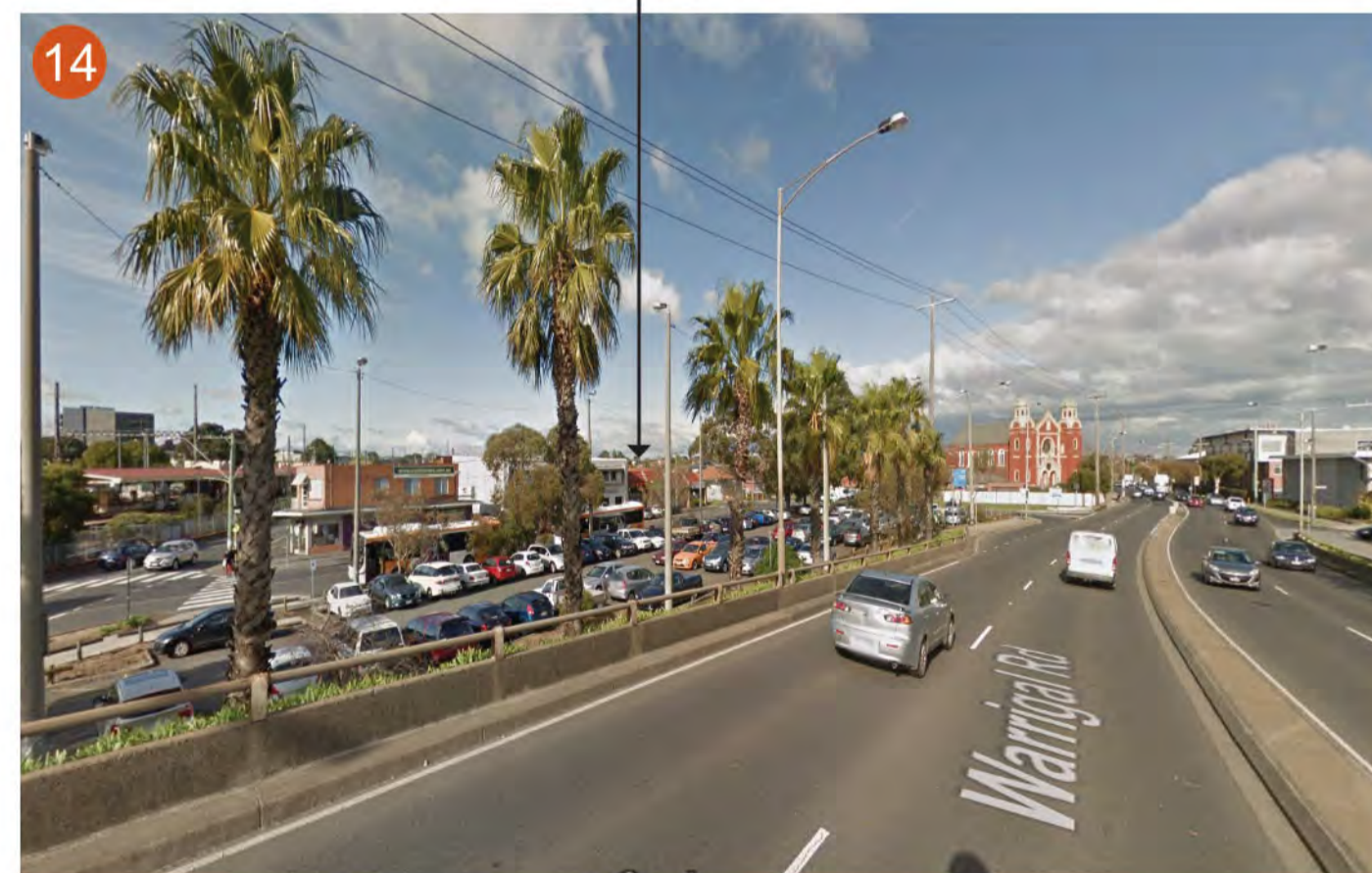
VIEW FROM WARRIGAL ROAD OVERPASS
