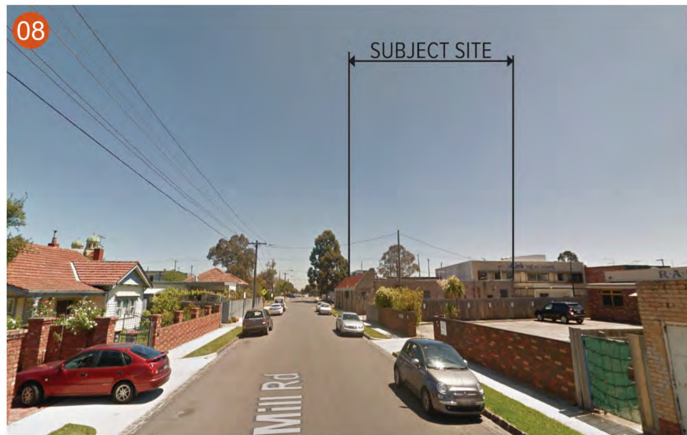
VIEW LOOKING WEST FROM MILL ROAD
