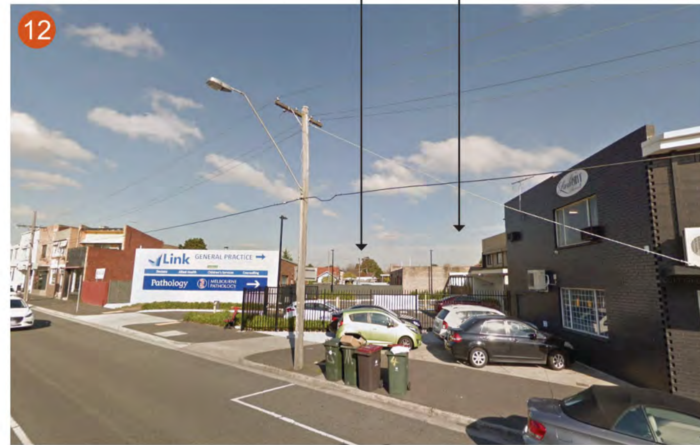
VIEW FROM HAUGHTON ROAD LOOKING SOUTH
