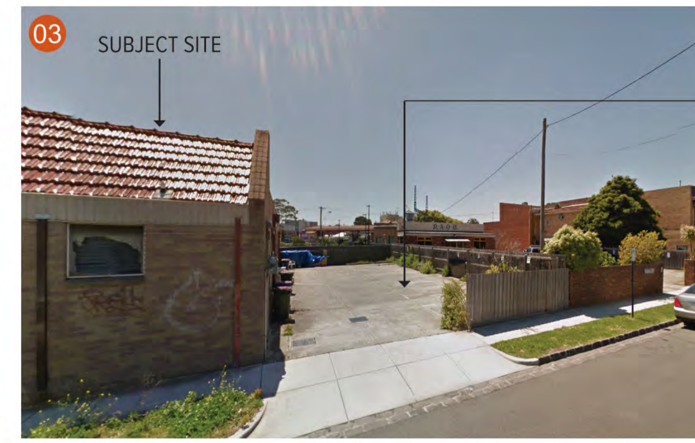
MILL ROAD - LOOKING NORTH OVER EXISTING CARPARK
