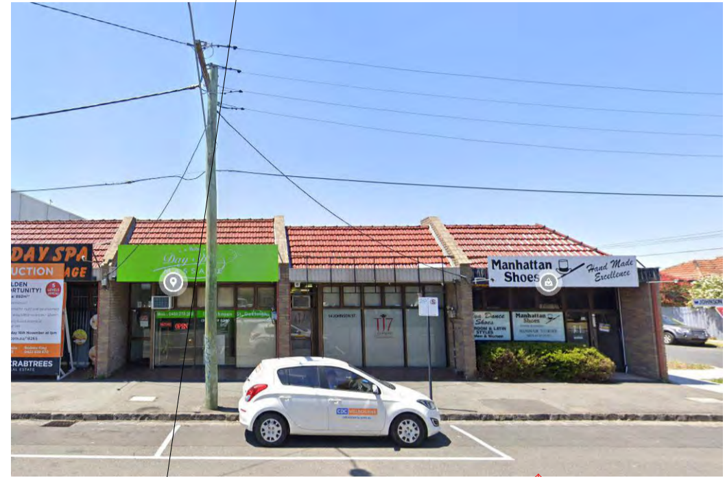
EXISTING SINGLE STOREY BRICK SHOPS TO BE DEMOLISHED
