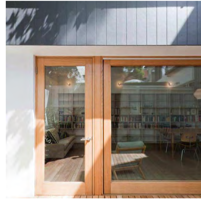
D01/D05 - TIMBER FRAMED ENTRY DOORS.
