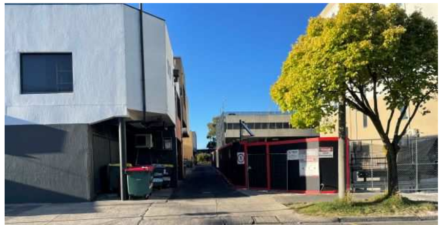
54 Montclair Ave - Proposed 11-Storey Mixed-Use Building under construction
