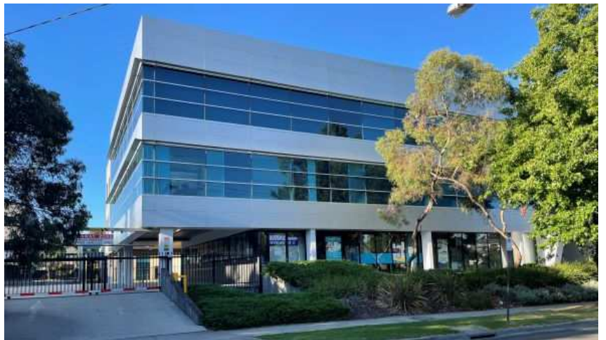
40-42 Montclair Ave - Existing 3 level office building
