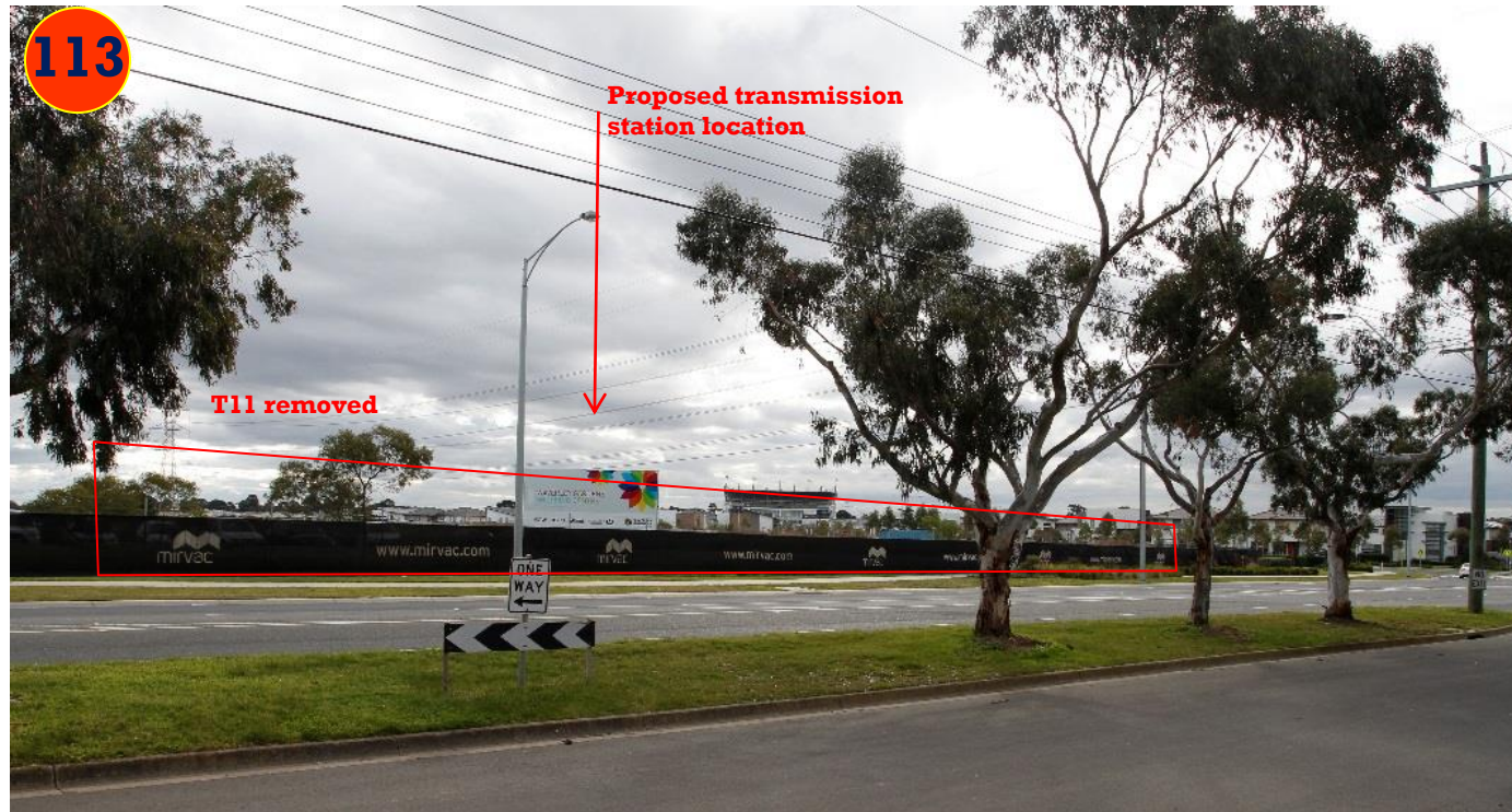
Figure 8 Photographic Analysis of the visual impact of the powerlines - underground powerlines (Endorsed 2.7.13 plans) view from the eastern side of Jacksons Road towards the review site
