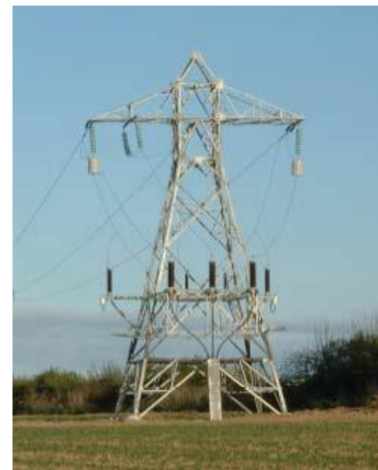
Figure 12 example of a 100kV tower and overhead lines being transitioned on the tower structure to cables that then go underground (images extracted from Professor A. Kalam report 1 August 2014).
