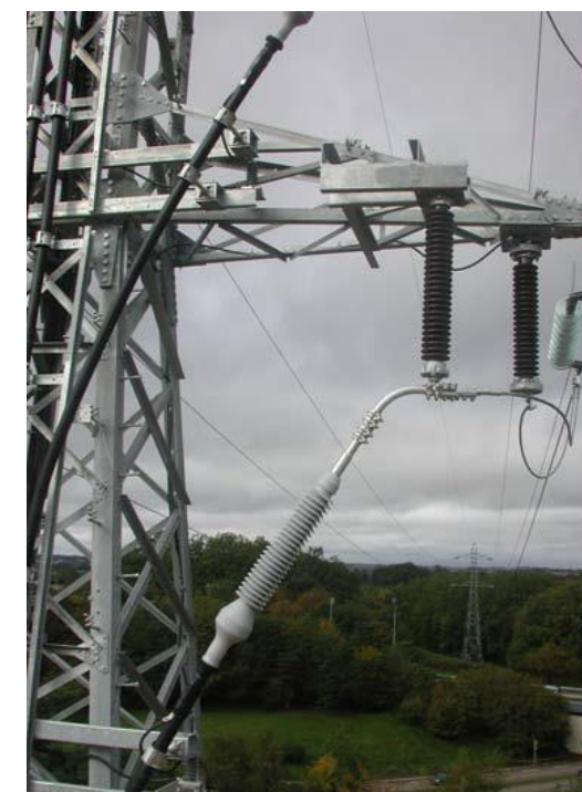
Figure 11 a & b examples of tower and overhead lines being transitioned on the tower structure (at 90kV) to cables that then go underground (images extracted from Professor A. Kalam report 1 August 2014).
