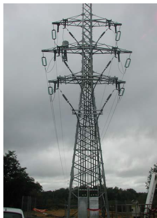
Figure 11 a & b examples of tower and overhead lines being transitioned on the tower structure (at 90kV) to cables that then go underground (images extracted from Professor A. Kalam report 1 August 2014).
