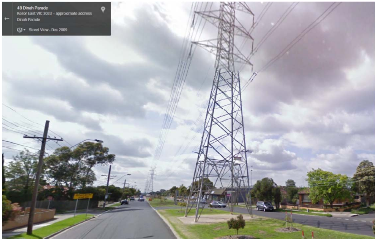
Figure 1 220kV Transmission Line Towers, Dinah Parade East Keilor, Victoria
