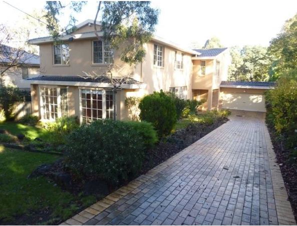
View to west from the entry into 39 Regent Street from Regent Street
