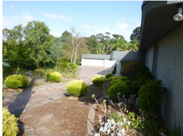
View to south west along the dwelling to the garage, showing the driveway and paving in 35-37 Regent Street
