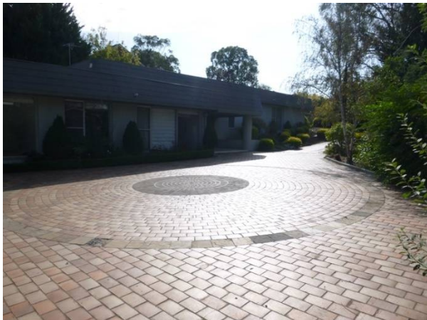
View to north-east over paved turning area showing relationship to the dwelling in 35-37 Regent Street
