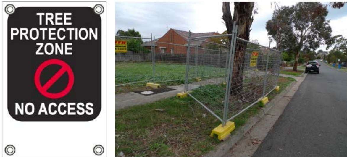
Figure 2: Example of signage for TPZ and of appropriate TPZ fencing.
