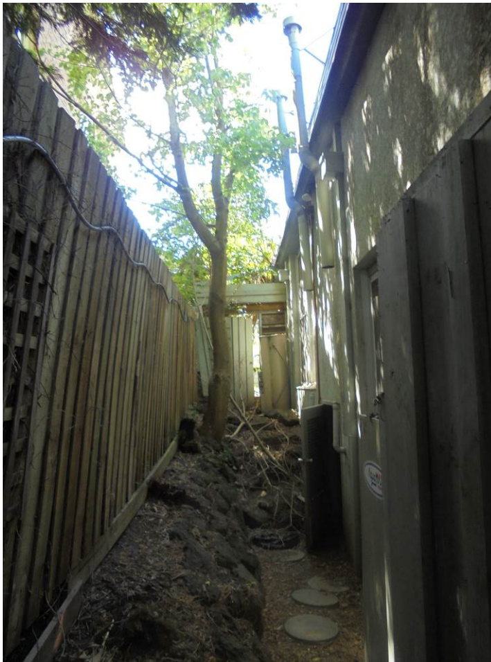
Figure 6: Shows the existing conditions along part of the northern boundary and tree 34, a Box Elder (Acer negundo). Where the alignment of the rock retaining wall is maintained within new designs, the impacts to the trees 33, 34 and tree group 4 would be minimal.
