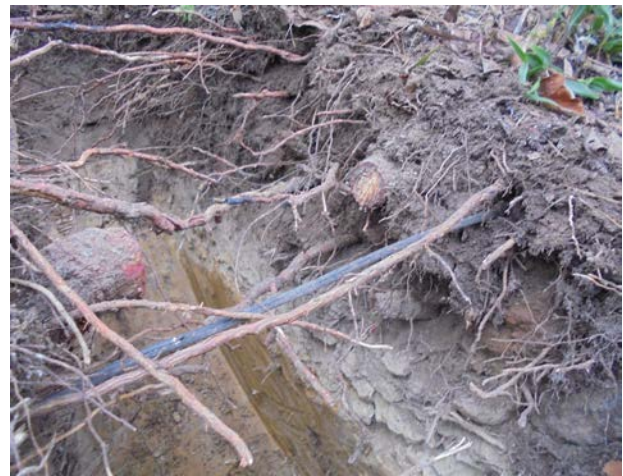
Above right: View to the east showing the southern trench alignment. No roots from the Lemon-scented Gum were noted within the trench alignment. Pink line indicates copper water or gas pipe.
