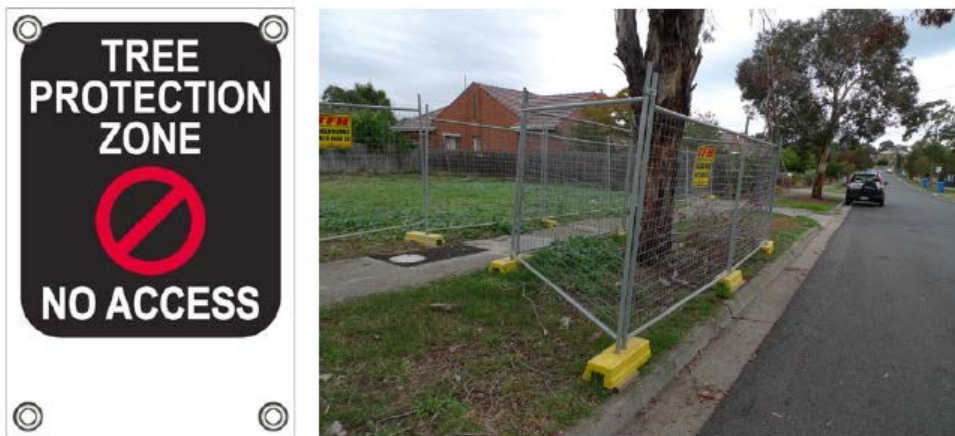
Figure 2. Example of tree protection fencing and signage for a street tree. This type of fencing is suitable for trees to be retained within the subject site.
