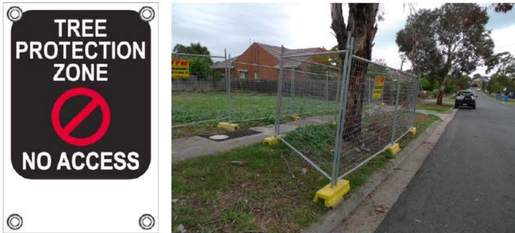
Figure 1. Example of tree protection fencing and signage for a street tree. This type of fencing is suitable for trees to be retained within the subject site.
