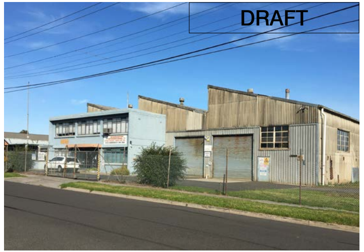
Older Industrial Built Form - Hargreaves Street
