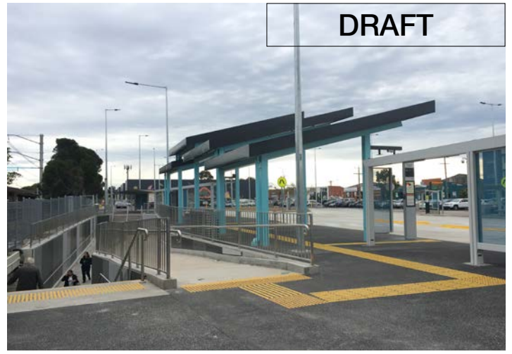
Huntingdale Station - Underpass Ramps & Bus Interchange Shelter
