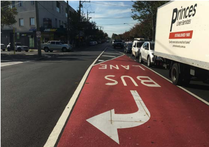
Bus Turning Lane Huntingdale Road
