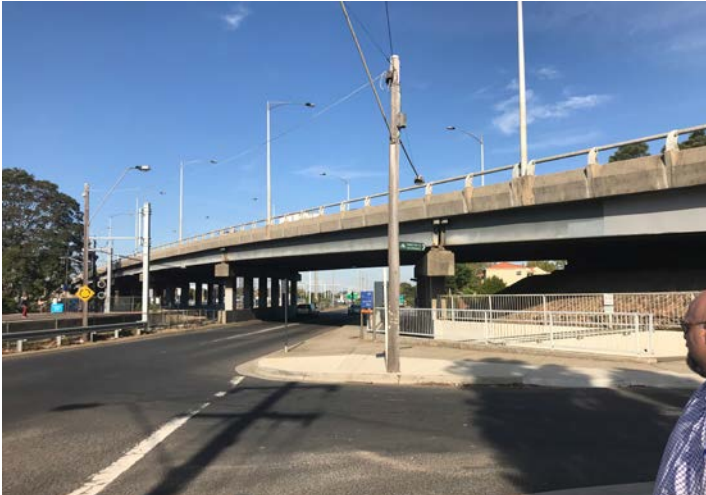
North Bridge - viewed from corner Haughton Road & North Road service lane
