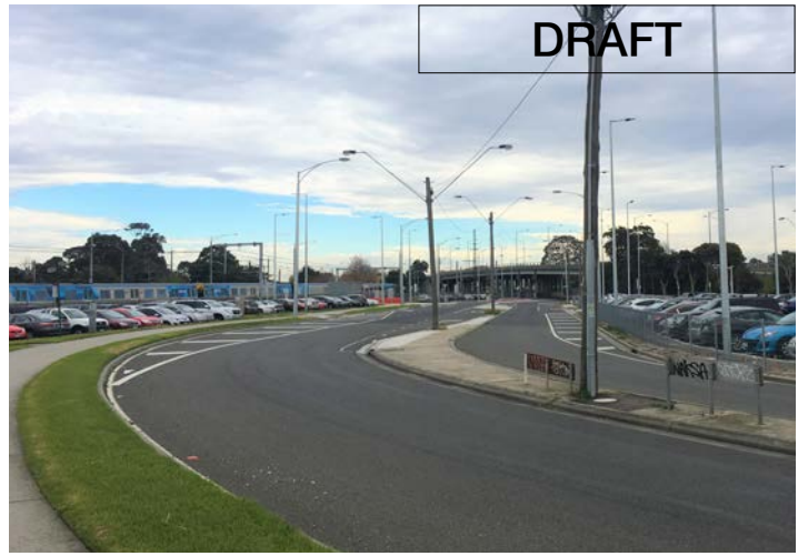
Huntingdale Station Car Park - North Road
