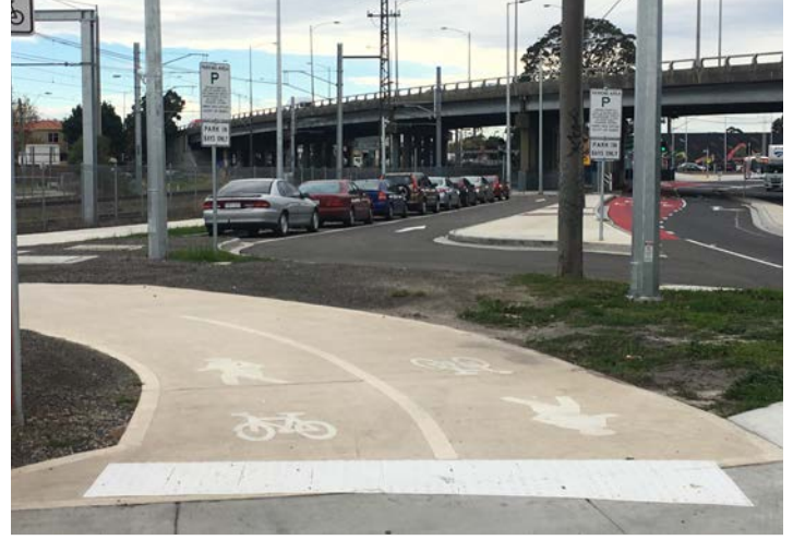
Rail Trail Connection between Huntingdale Station and North Road
