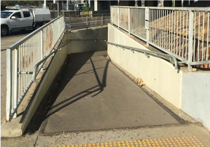
Huntingdale Station Underpass - Haughton Road
