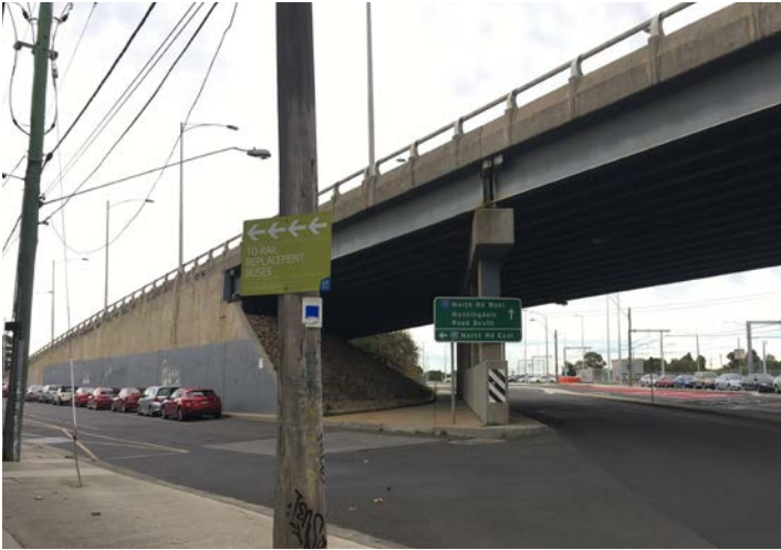
Poor Pedestrian Amenity - North Road
