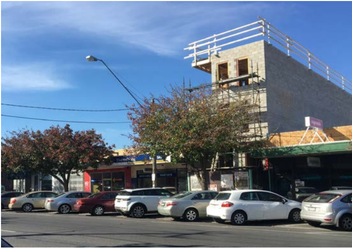
3 Storey Mixed Use Development at 302 Huntingdale Road
