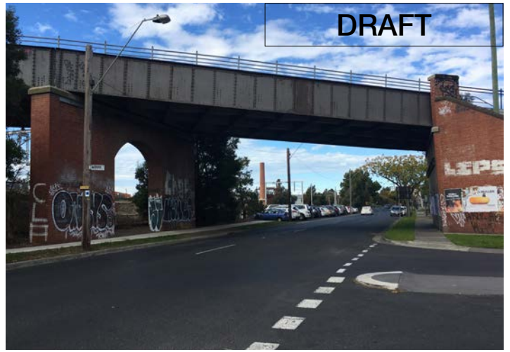
Hanover Street Bridge & Boiler House Stack
