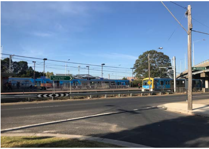
Huntingdale Station - viewed from Haughton Road
