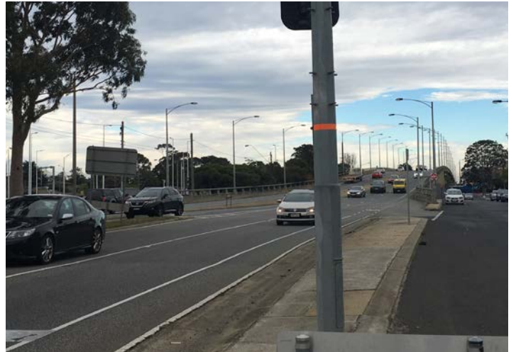
North Road Overpass
