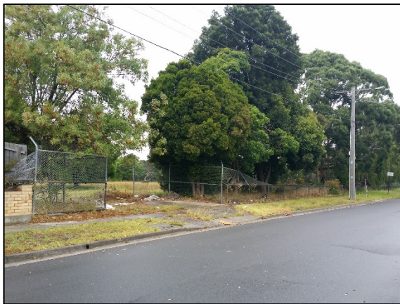
Alvina Street frontage view south-east
