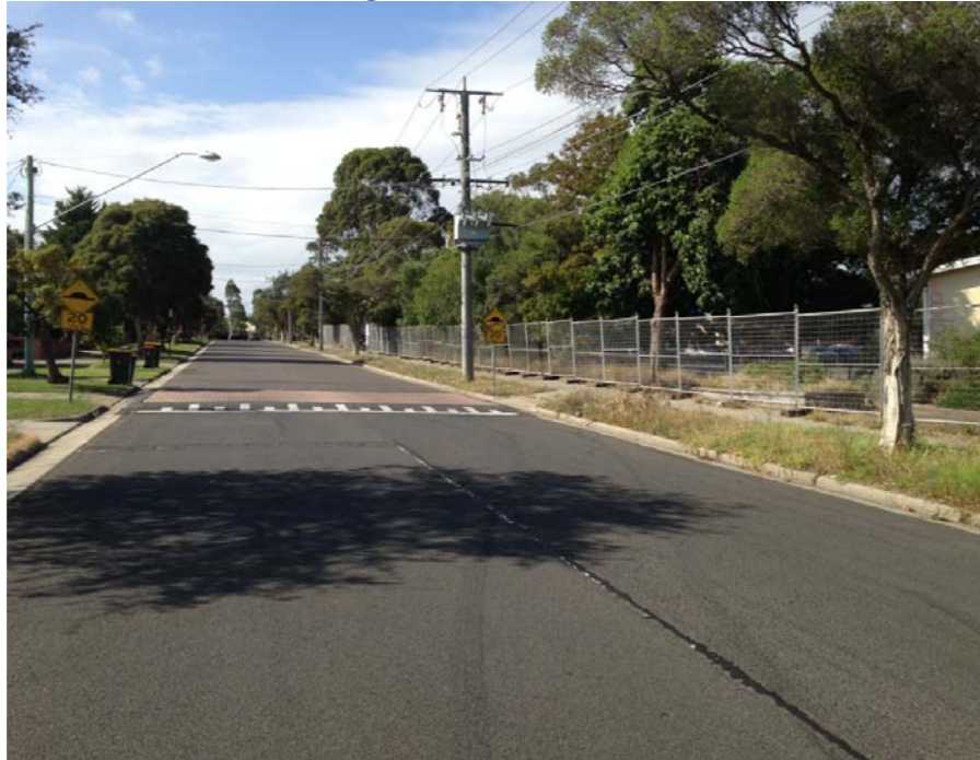
Photo 2-2: Browns Road looking north
